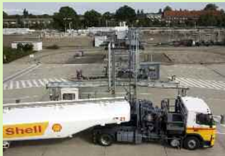
The tank farm fulfills all safety standards
