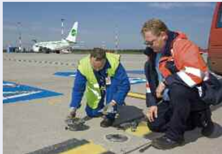
Apron lighting check
