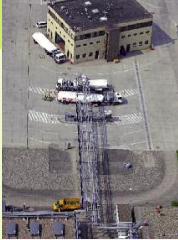
The central kerosene store is subject to strict security provisions.
