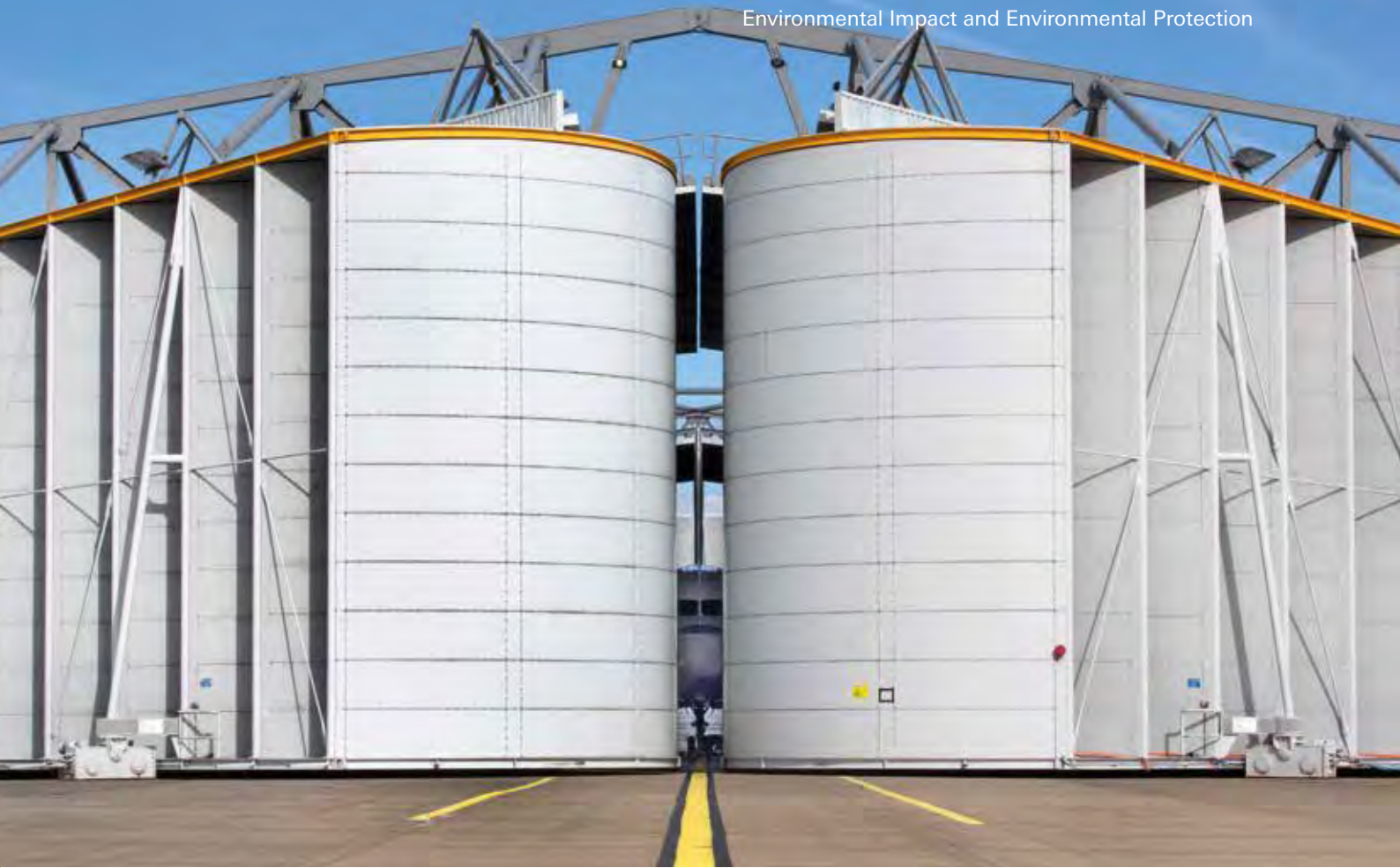
The Noise Protection Hangar, designed and constructed by FHG, offers effective protection against noise generated by engine test runs.
