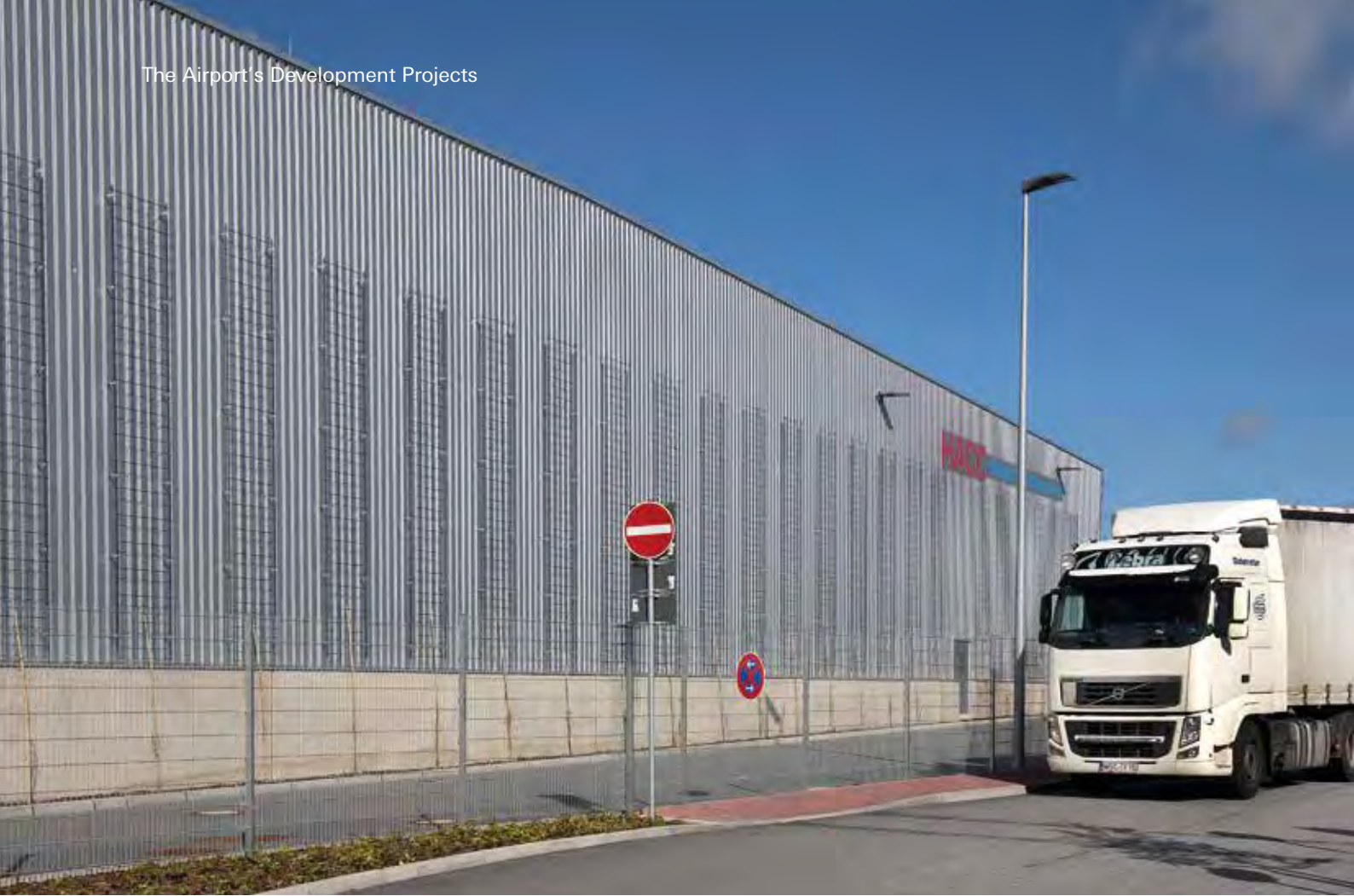
Entering service in 2016, the new Air Cargo Center fulfils all current sustainability standards.
