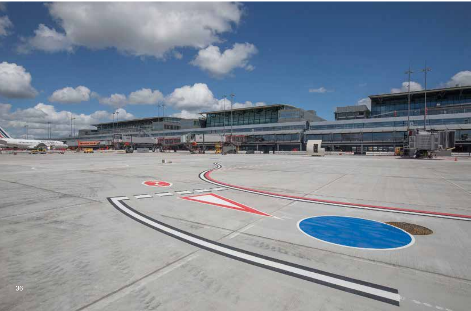
Apron 1 is being comprehensively refurbished.
