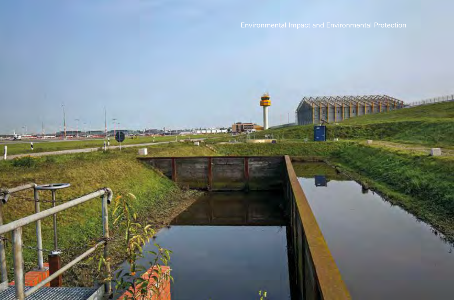
A total of nine rainwater retention basins protect Tarpenbek from any contamination that may occur.
