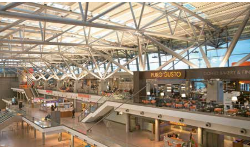
As well as the terminals, Hamburg Airport operates a large number of other buildings with various functions
