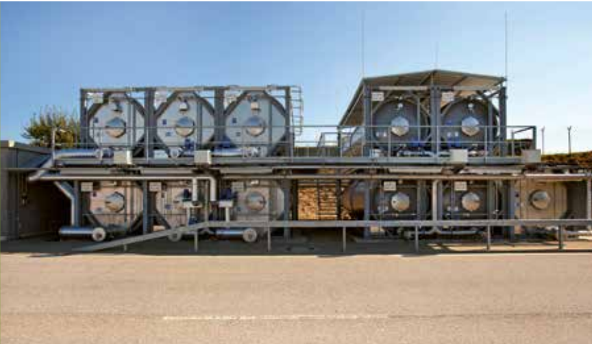
The de-icing agent storage was recently completely overhauled
