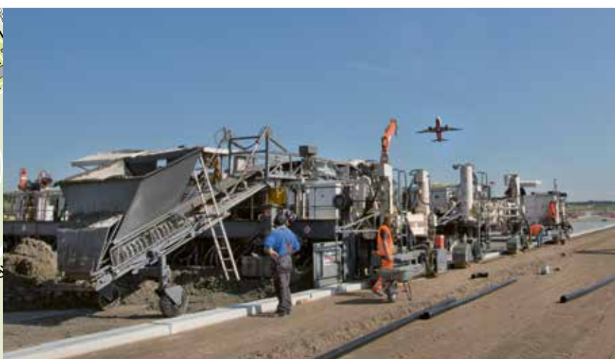
Initial work in the apron 1 south area
